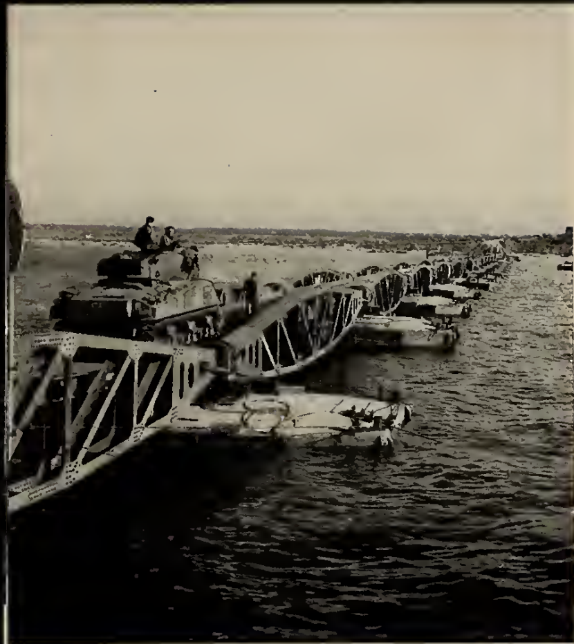
11. The floating roadway is completed, and a tank starts across.
